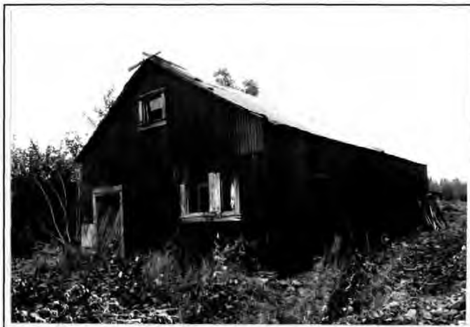
Figure 36. The Donnelley and Sheppard Cold Storage Building, 1993. The view is looking southwest.
